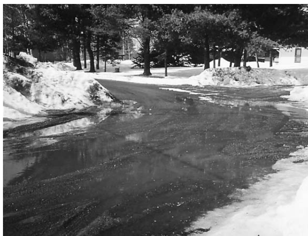
As spring thaw weakens pavements, trucks carrying heavy loads can damage them.
